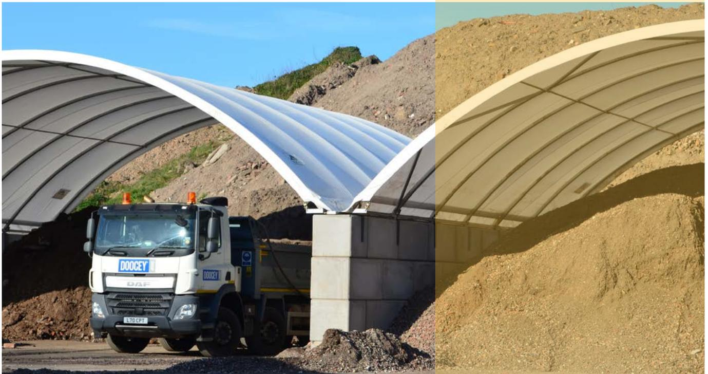
Doocey's plan was to build three new Zappshelters, these covered areas were to be used to store recycled construction & demolition waste and utility excavation arisings.
