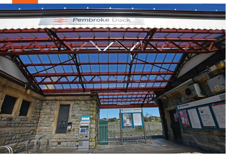
Pembroke Dock are designed to allow access from underneath, rather than on top of the roof, enhancing the safety of the roof. These access hatches are also designed to blend into the glazing and fit the heritage requirements of this historic station.
